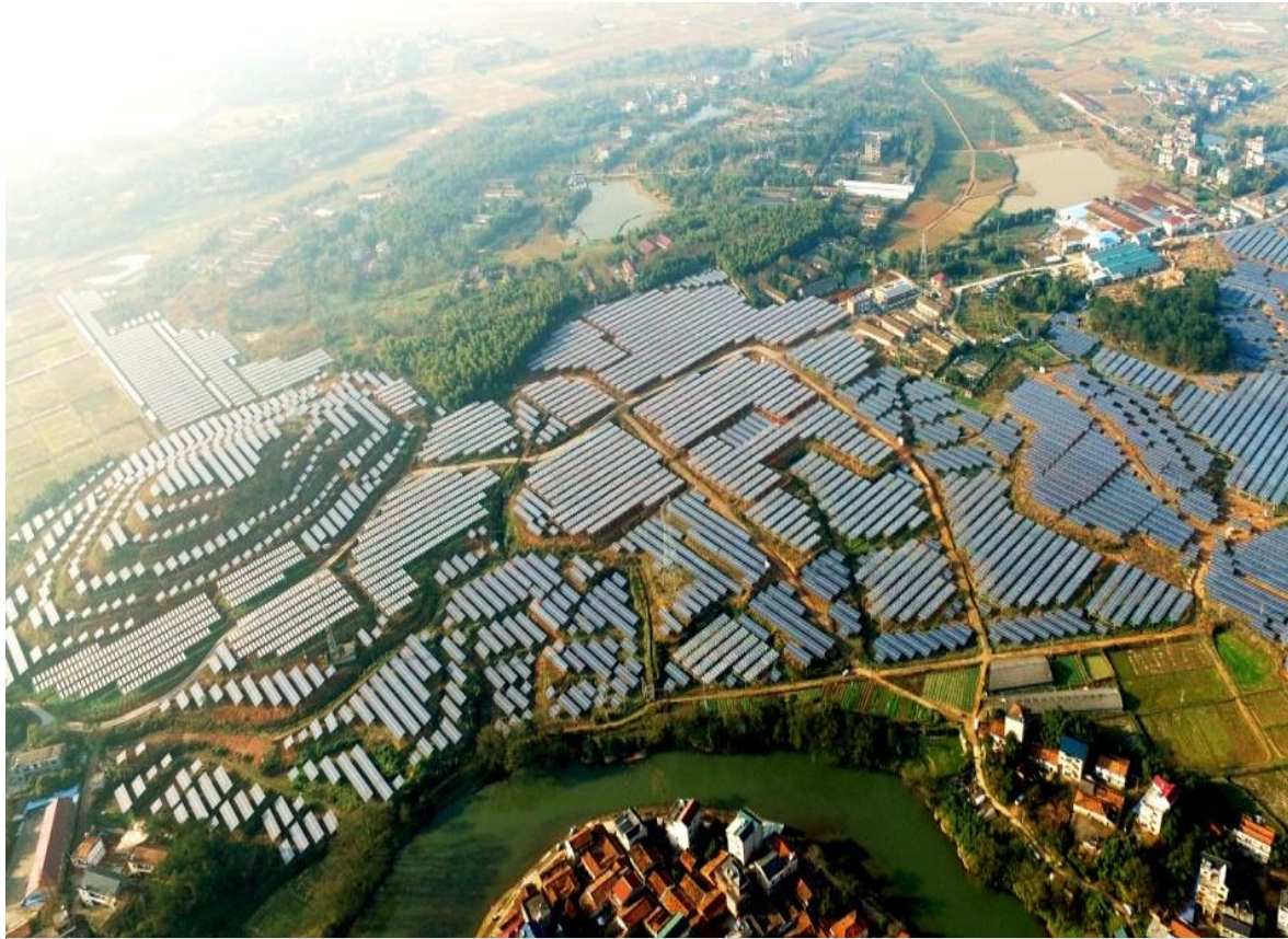
Jiangshan FIRST 15.19MWp Agricultural (forest) light complementary photovoltaic power station project
